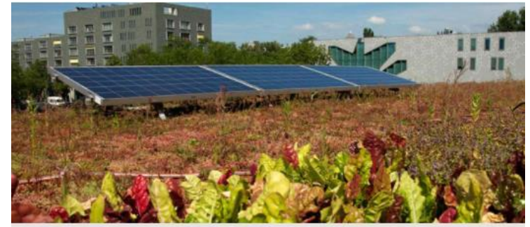
Combined with solar panels
